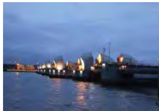
Thames Barrier, image courtesy of Atkins
