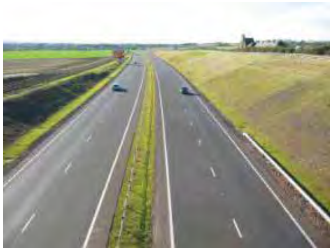
Carriageways, image courtesy of Atkins
